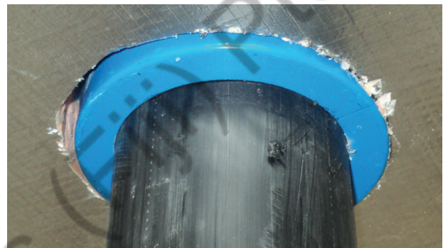
Figure 7 Penetration example - Kingspan Kooltherm ® K10 G2 Soffit Board installed tight around the fire collar and HDPE service pipe.
