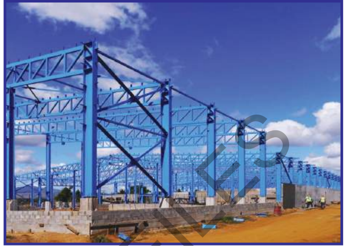
Motibhai Business Park Floor Area = 10,000m 2 Kings Road, Legalega, Nadi
