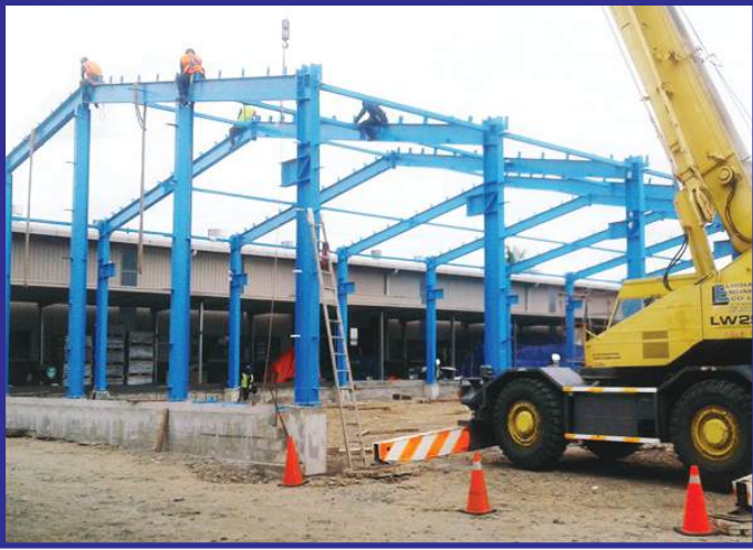
Roofing and Profiles Factory Floor Area = 1,000m 2 Kings Road, Yalavevu, Ba.
