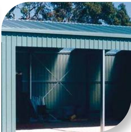
Open Bay Garage
