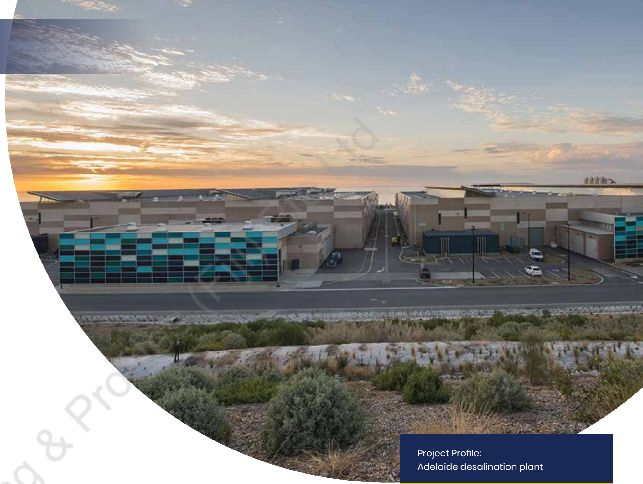
Adelaide desalination plant. Hurricane HI
