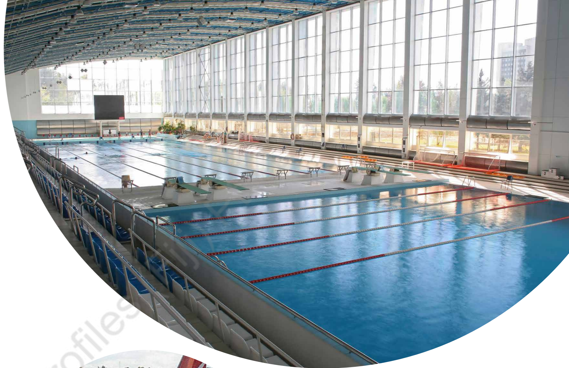
Hurricane® was installed in indoor swimming centres to reduce condensation and humidity.
