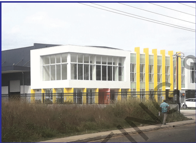
UB Freight Warehouse Floor Area = 2000m 2 King Road, Natabua, Lautoka.
