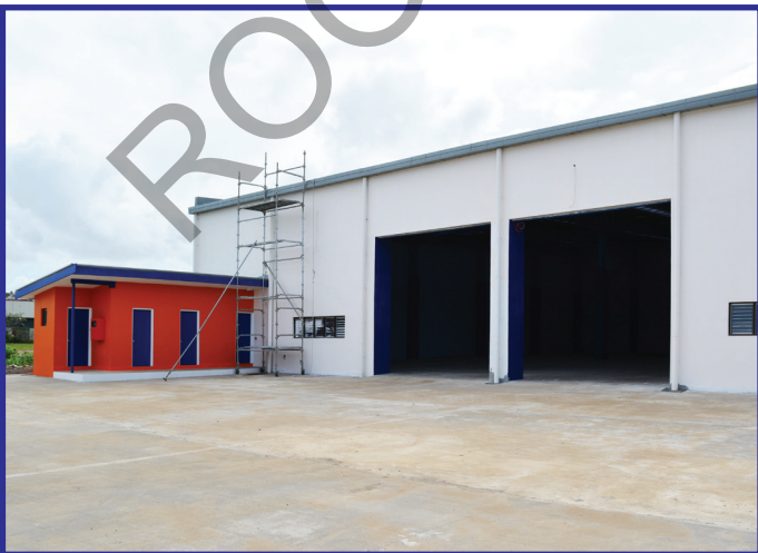
R.C Manubhai Yard 5 Floor Area = 2000m 2 Carpenter St, Raiwaqa, Suva.
