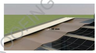
Overlap by 50 mm at joins and apply 72 to 100 mm reinforced foil tape to top of join. Alternatively allow 150mm overlap when joins are not to be taped.
