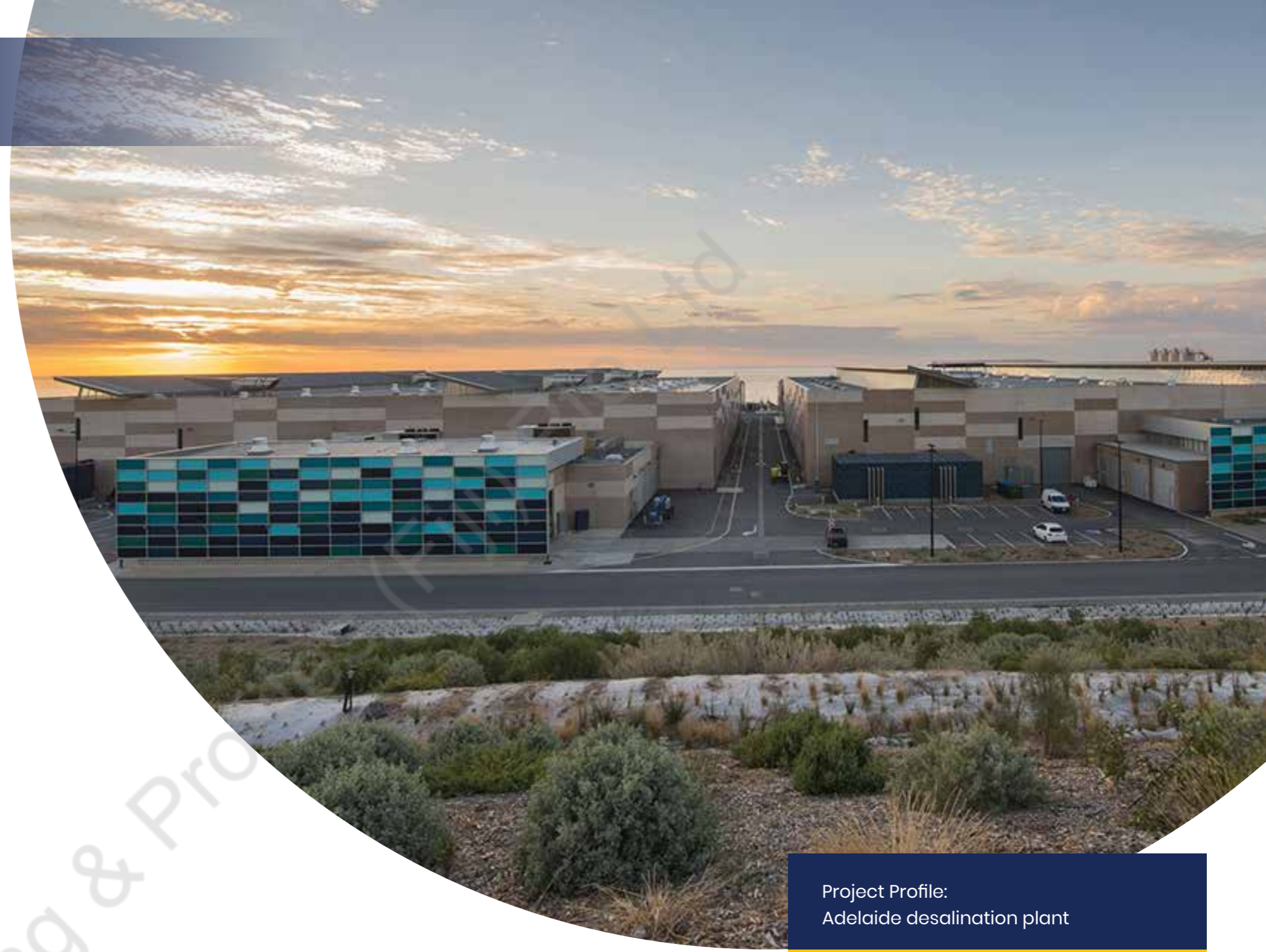
Adelaide desalination plant. Hurricane HI
