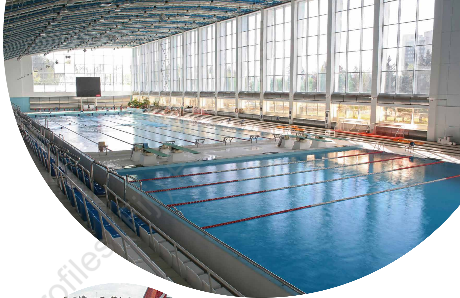
Hurricane® was installed in indoor swimming centres to reduce condensation and humidity.
