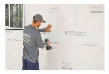
Recommended for cooler regions to help manage condensation. It allows vapour to escape the building, whilst helping stop vapour, water, and wind from entering.
