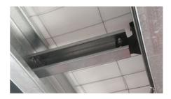
A C Section purlin can be placed between purlins to form the brace
